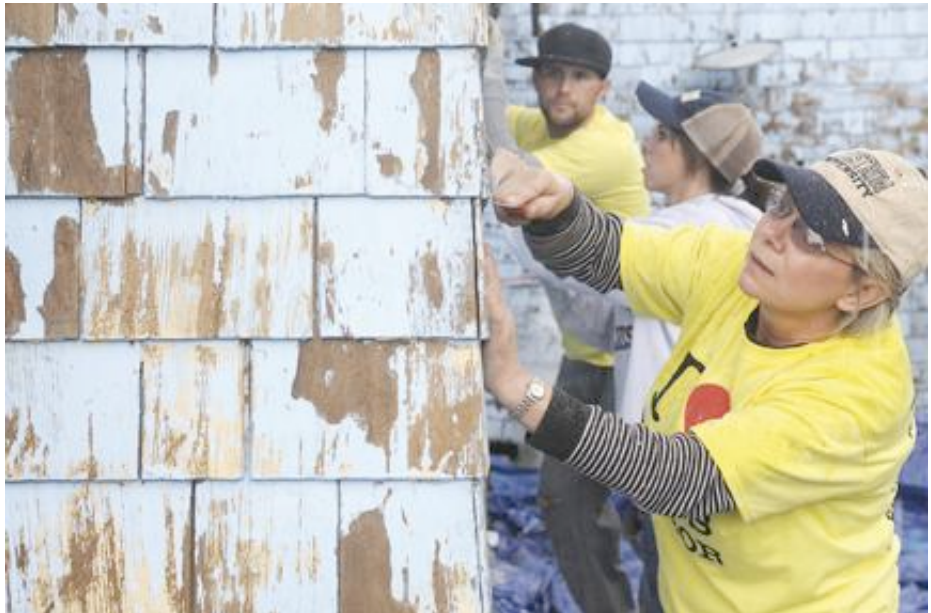
MACLEOD PAPPIDAS | THE DAILY WORLD Volunteers Celia Barry, right, her daughter Traci Barry and Noah Gardiner scrape old paint off a house on the 2900 block of Simpson Avenue in Hoquiam as a part of the Paint the Corridor project Saturday morning. Due to rain, work was diverted from painting houses to prepping them for painting at a future date.
